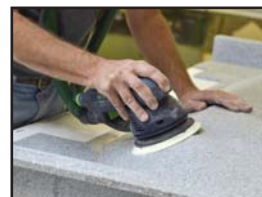
Final buffing and finishing onsite during installation
